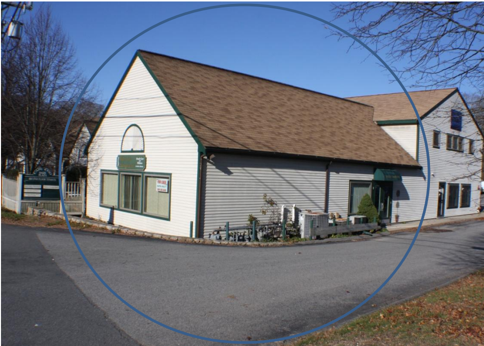
Closer view of Unit #16
