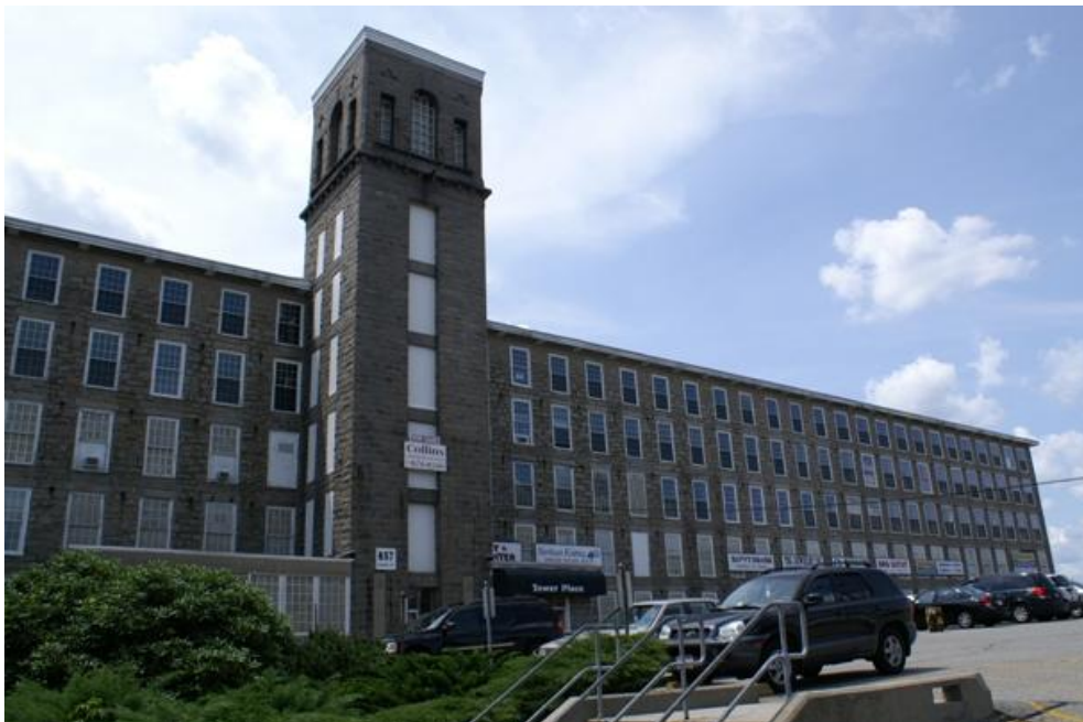
Exterior of Building
